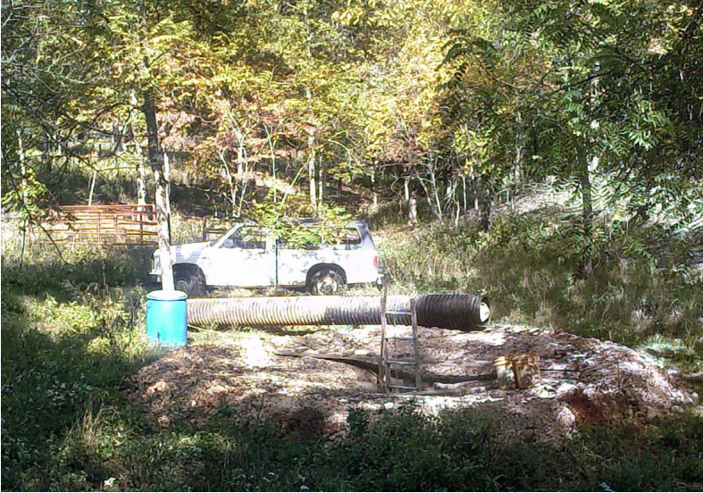
The hole is 20' 8" deep. The culvert is 20' long. The barrel is a 55 gallon plastic barrel for recharge.
