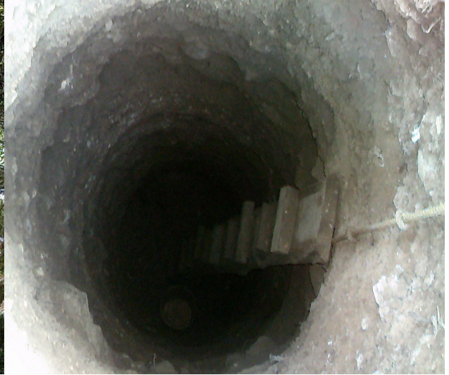
The hole is 20' 8" deep. The culvert is 20' long. The barrel is a 55 gallon plastic barrel for recharge.
