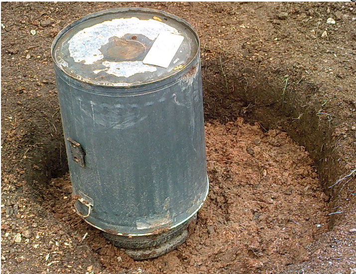
The hole is sealed with 2' of clay I dug from deep in the hole. I put it on top to keep the surface water out.
