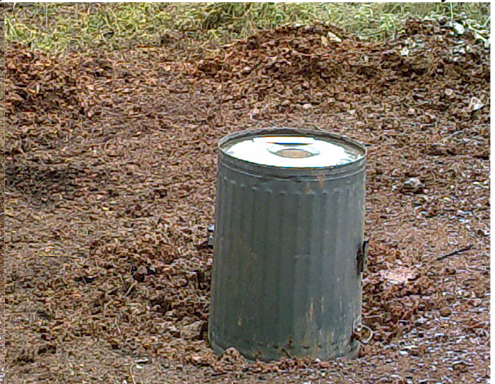
The hole is sealed with 2' of clay I dug from deep in the hole. I put it on top to keep the surface water out.
