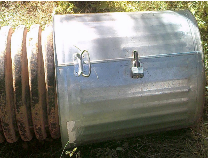
The galvanized can is pinned and locked onto the culvert. The culvert is inserted into the top of the barrel. The barrel has 4" of concrete and rock in the bottom for protection, and is set in sand (nylon felt covers holes). The hole was backfilled with 10' of rock above the 55 gallon barrel, and then with sand, dirt and then clay.
